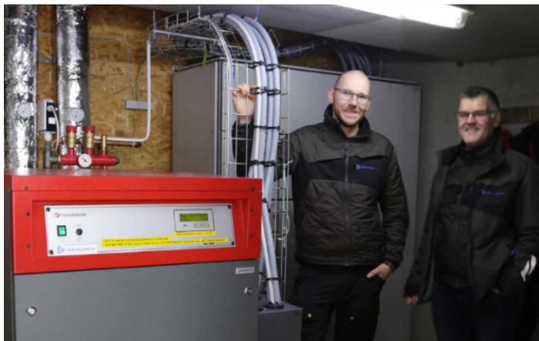
Figure 8: Deployment of an electric boiler at Hotel SØMA in Nuuk, replacing fuel oil and reducing CO 2 emissions by 142 tonnes annually (Nukissiorfiit, 2024b)
