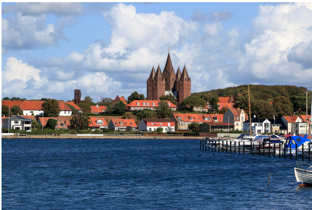
Kalundborg is one of the municipalities that can expect a large bill per capita in relation to future flooding
